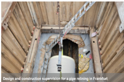
Design and construction supervision for a pipe relining in Frankfurt
