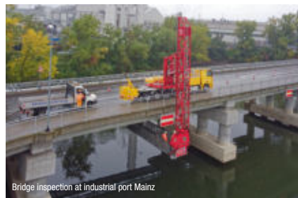
Bridge inspection at industrial port Mainz
