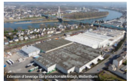
Extension of beverage can production site Ardagh, Weidenburg
