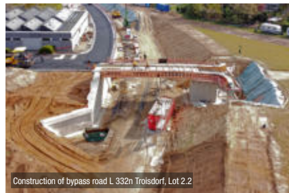
Construction of bypass road L 332n Troisdorf, Lot 2.2
