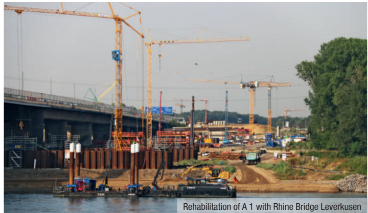
Rehabilitation of A 1 with Rhine Bridge Leverkusen
