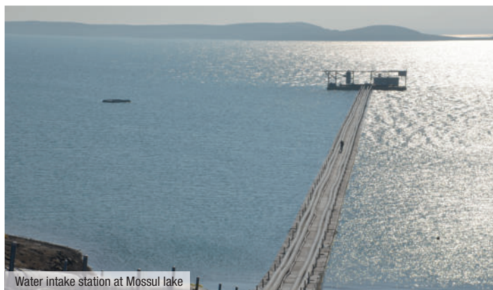
Water intake station at Mossul lake
