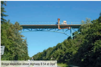
Bridge Inspection above Highway B 54 at Olpe
