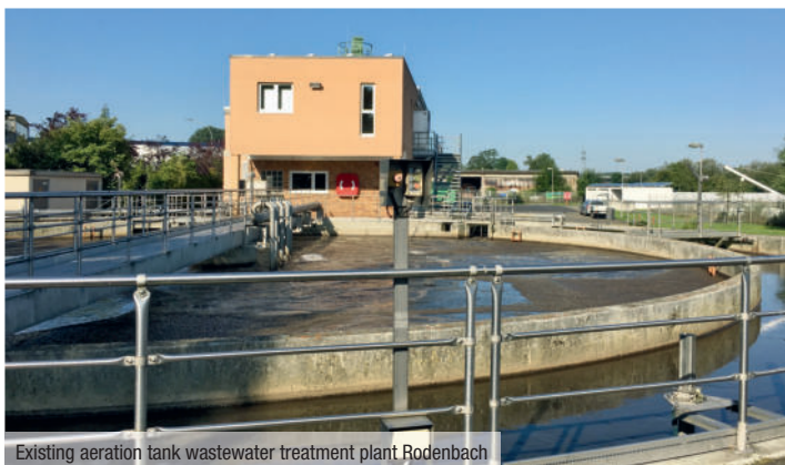
Existing aeration tank wastewater treatment plant Rodenbach
