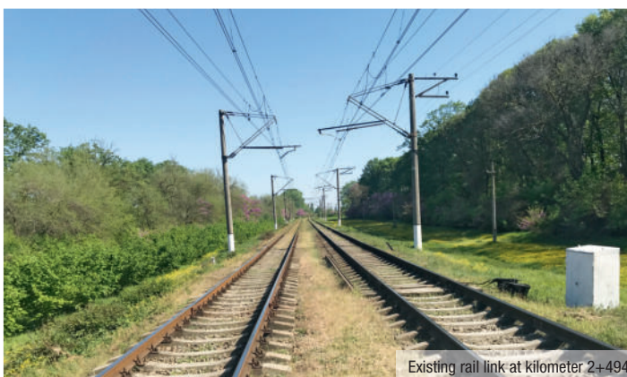
Existing rail link at kilometer 2+494
