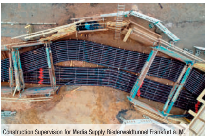
Construction Supervision for Media Supply Riederwaldtunnel Frankfurt a. M.
