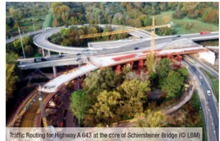
Traffic Routing for Highway A 643 at the core of Schiersteiner Bridge (© LBM)
