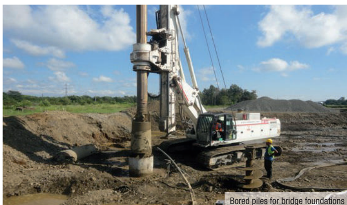
Bored piles for bridge foundations
