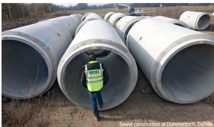
Sewer construction at Dümmerbach, Datteln
