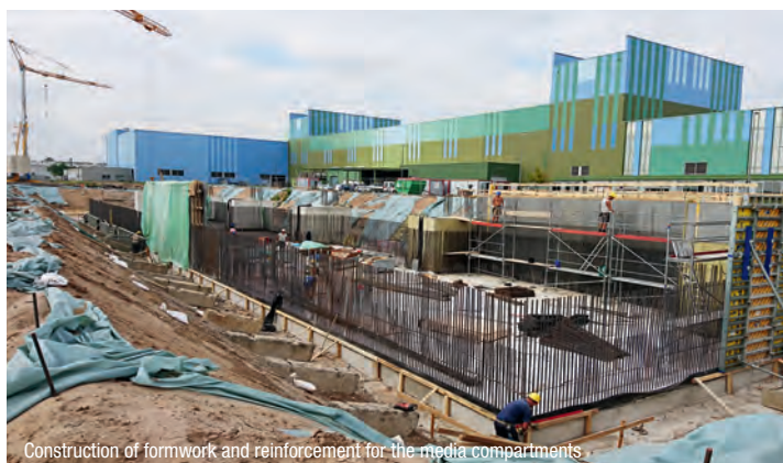
Construction of formwork and reinforcement for the media compartments
