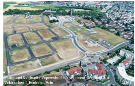
Design and Construction Supervision for Development of Building Area Schänzchen III, Hochheim/Main
