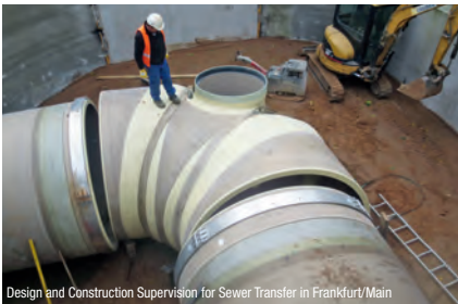
Design and Construction Supervision for Sewer Transfer in Frankfurt/Main
