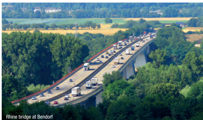
Rhine bridge at Bendorf
