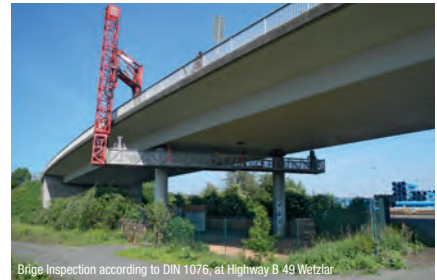
Bridge Inspection according to DIN 1076, at Highway B 49 Wetzlar
