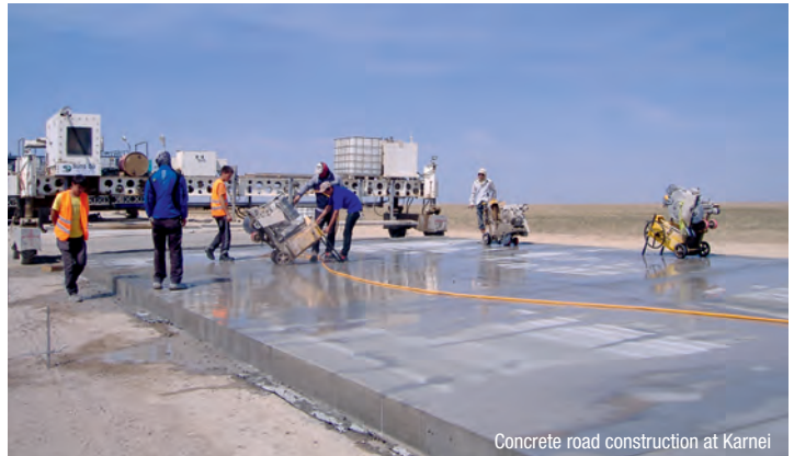
Concrete road construction at Karnei
