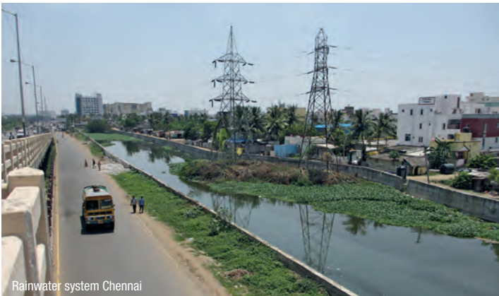
Rainwater system Chennai
